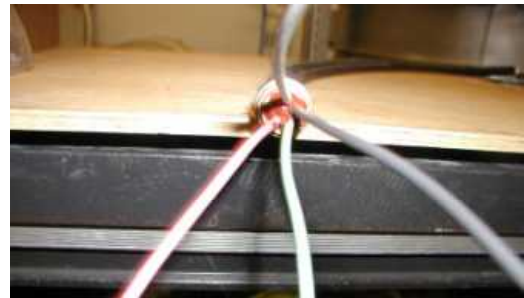
Figure 36 Epoxy Compound Packed Around
